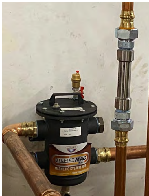
Activflo installed with a Zilmet Magpro in a bypass loop of a closed system
