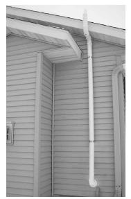
**Figure 10** Vent Line Installation (3 inch)
